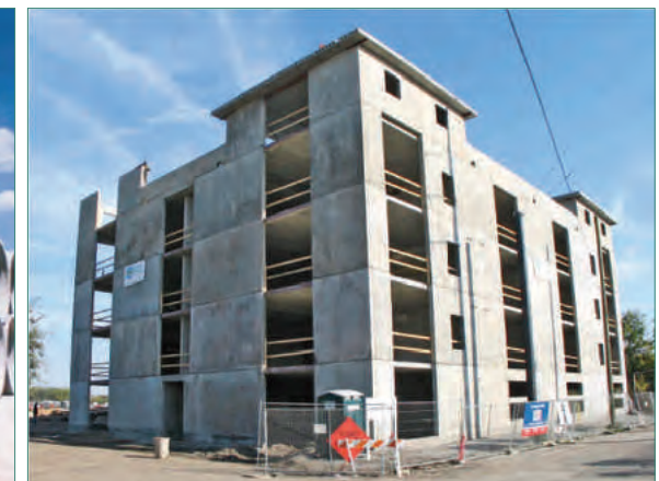
Precast Wall Panels
